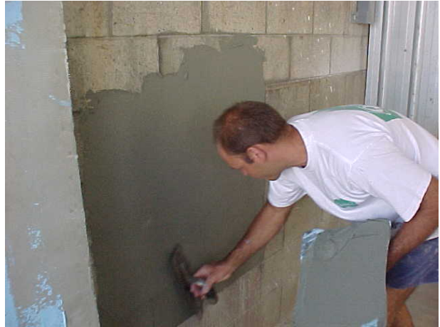
2. Apply High-Build SKIMCOAT
