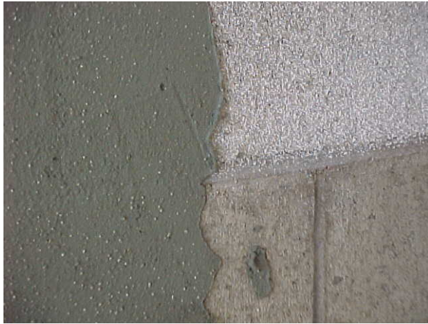
3. High-Build SKIMCOAT closeup
